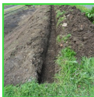
Fig 2: Excavate anchor Trenches
