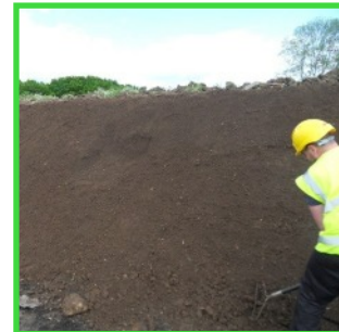
Fig 6: Rake in 10mm cover of friable topsoil
