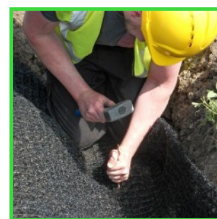
Fig 3: Pin GeoMat into Anchor Trench
