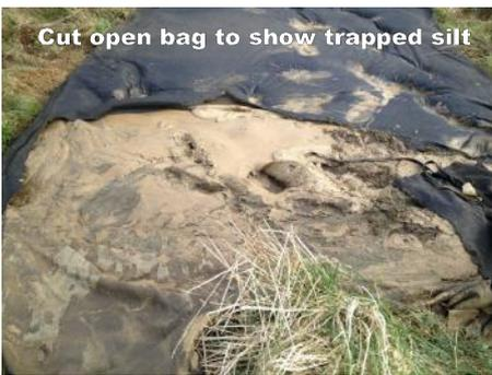
Hy-Tex Ultra Dewatering Bags provide an effective way to collect harmful sediments from dirty water pumped out of excavation works (such as foundations, pipe line construction, water, sewer and utility trenches, waterways and lakes) that would otherwise pollute the surrounding environment.
