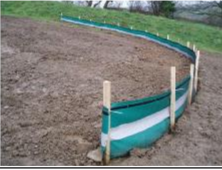
Hy-Tex Terrastop silt fence in use on National Grid's Felindre to Brecon gas pipeline project
