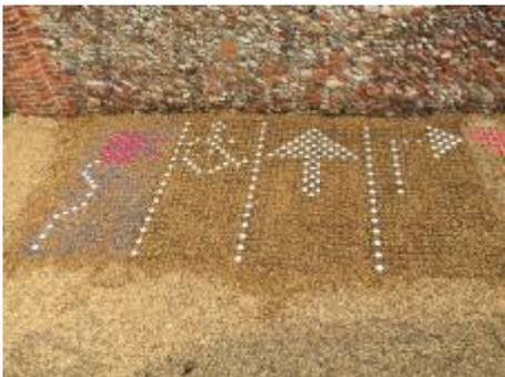
**Hy-Pave Dura** porous cellular pavers are strong, interlocking, plastic tiles used to create permeable reinforced grassed or gravel areas for a variety of applications, both domestic and commercial, providing an environmentally friendly alternative to tarmac or concrete.
