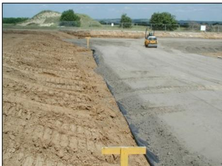
**The extremely popular Hy-Tex Terralys™ LF 16/16 is fully compliant with the Department of Transport Clause 609 specification requirements, and is recommended for general earthwork and road-base separation applications.**
