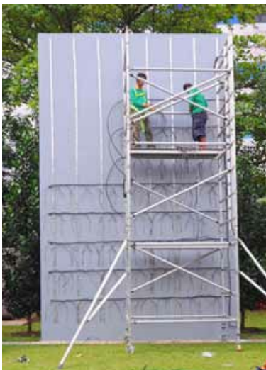
Installation of VGM®
