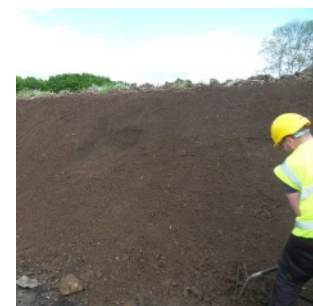
Fig 6: Rake in 10mm cover of friable topsoil
