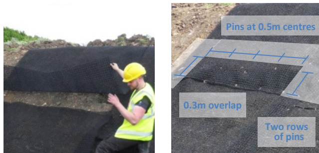
Fig 8: Cross-slope overlaps and pinning
