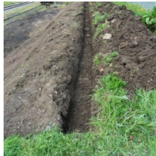
Fig 2: Excavate anchor Trenches
