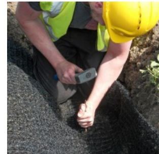
Fig 3: Pin GeoMat into Anchor Trench
