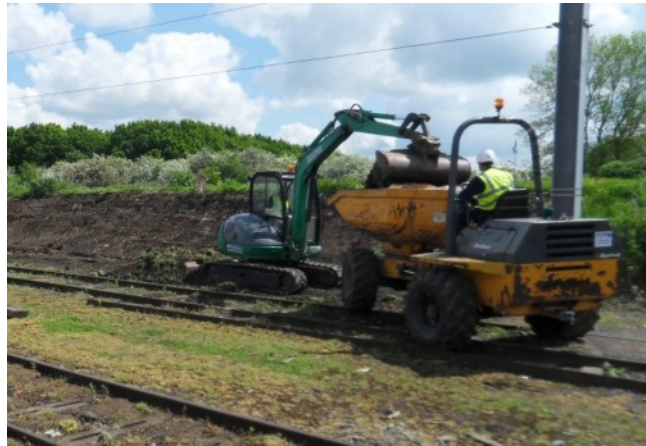
Fig 1: Prepare slope to create even surface
