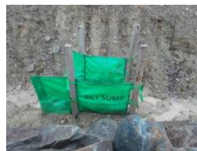
2. Secure Silt Sump with 6 posts
