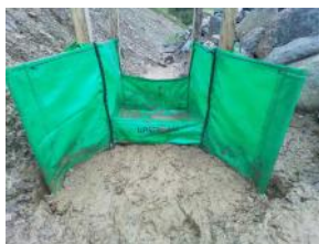
4. Pack soil and grass around wings/sides to create seal.
