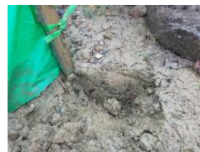
3. Dig in and bed in wings on both sides
