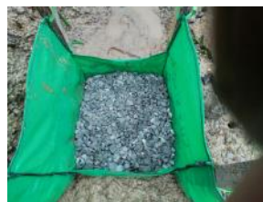
5. Add 20kg of 40mm clean aggregate and spread in base
