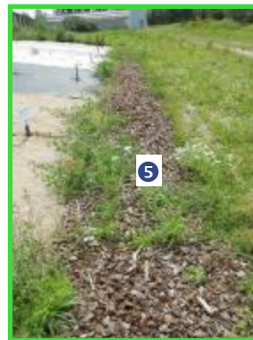
5. 10cm layer of bark chips used in front of slope.
