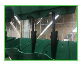
Where two sheets of Unistrut butt up to each other one mesh clip is sufficient to connect and support both.
