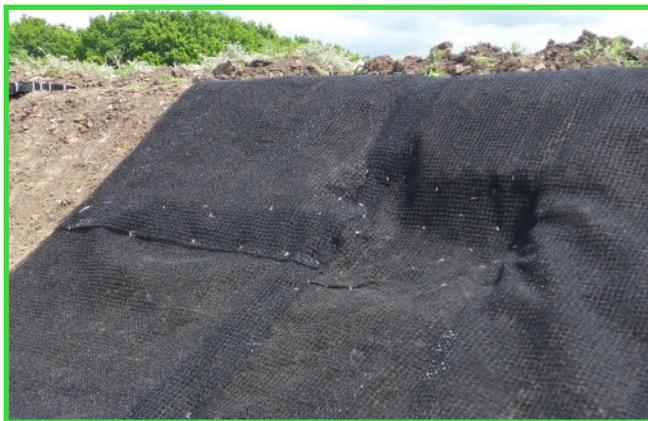
Fig 5: Ensure GeoMat is in intimate contact with the ground IN ALL PLACES
