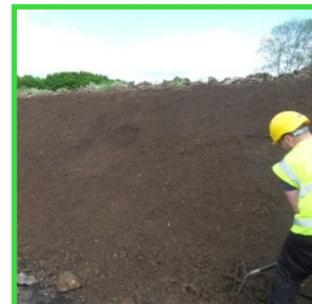
Fig 6: Rake in 10mm cover of friable topsoil
