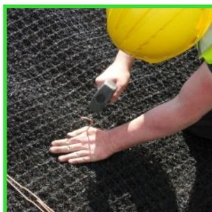
Fig 4: Pin GeoMat to slope
