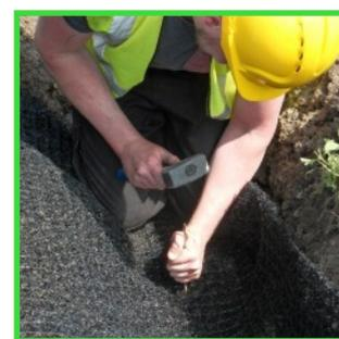
Fig 3: Pin GeoMat into Anchor Trench
