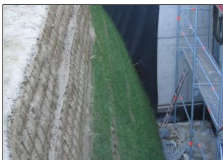
*GrassMat™ Supreme* is a new biodegradable textile, pre-sown with seed and fertilizer, which provides an easy method for effective vegetation restoration and erosion control on wide variety of landscapes from lawns to steep slopes.
