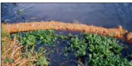
Hy-Tex *CoirLog* and *CoirPallet* biodegradable, coconut fibre bio-roll and mattress substrates work in harmony with nature, to protect and support banks, and shorelines, while promoting restoration of wetland environments.
